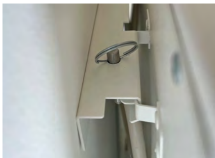
5. Insert the safety splints
