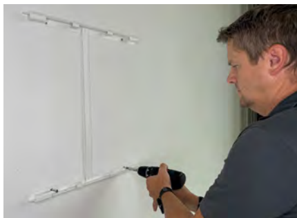
2. Drill the holes & secure the mounting bracket
