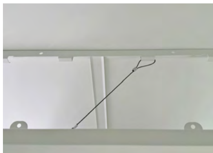
4. Hook on the safety cable & make the electrical connection
