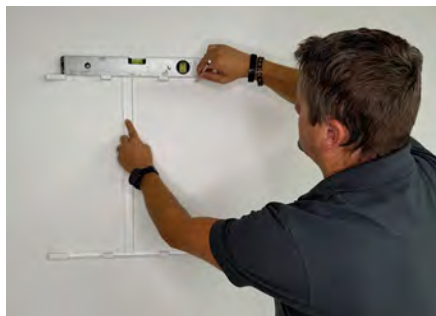
1. Mounting bracket acts as drilling template
