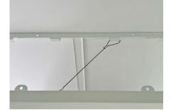
4. Hook on the safety cable & make the electrical connection
